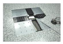
Remove first-piece tile by using one-cup or two-cup access floor lifter
